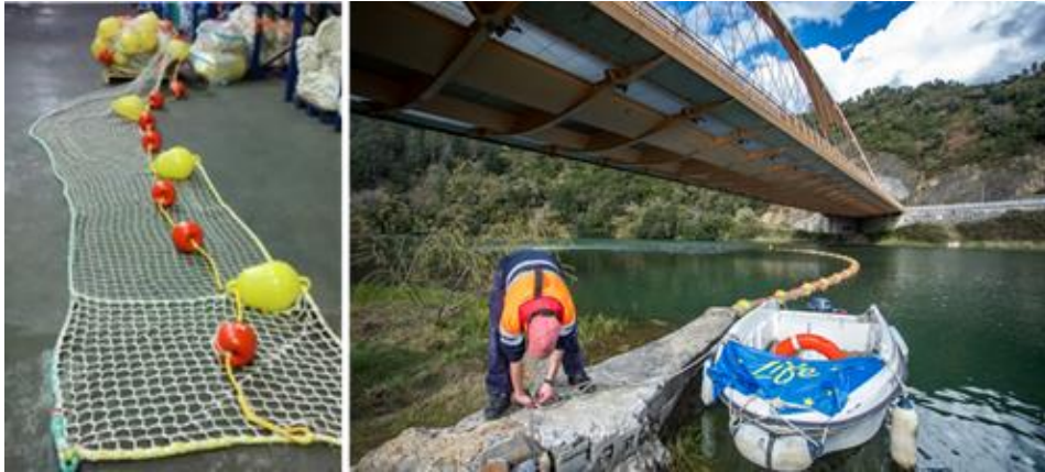
Figure 10 : Barrier (left) installed in Deba river (right)
